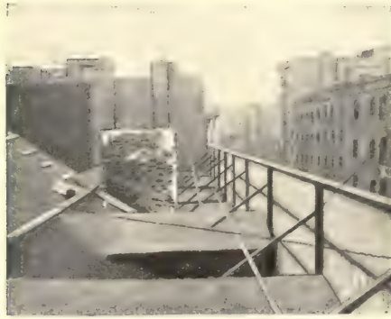
FIG. 102.—Advertising sign constructed in front of the only windows of six rooms, shutting out all light and air.
